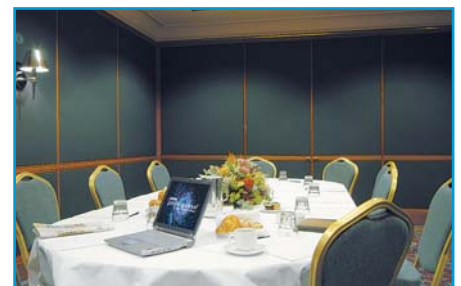
Each function room received a data communications upgrade to facilitate internet and email access and video conferencing.
